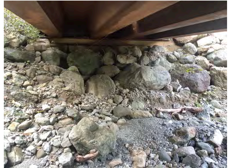
Left Bank Abutment when facing downstream
