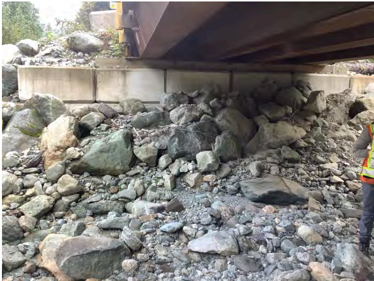
Right Bank Abutment when facing downstream
